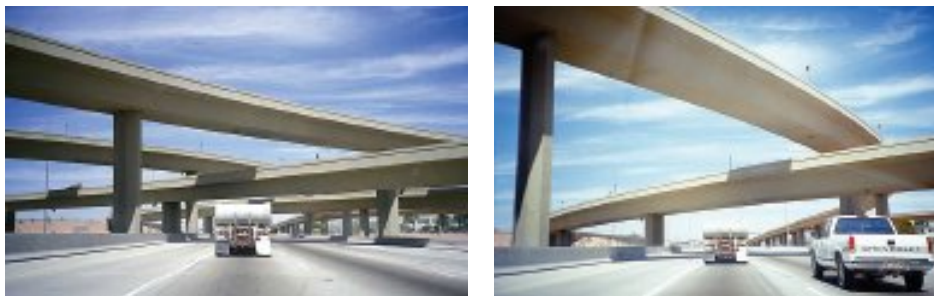
○ Figura VIII.3 y VIII.3 bis. Autopista interestatal Freeway 15, Phoenix, USA.
